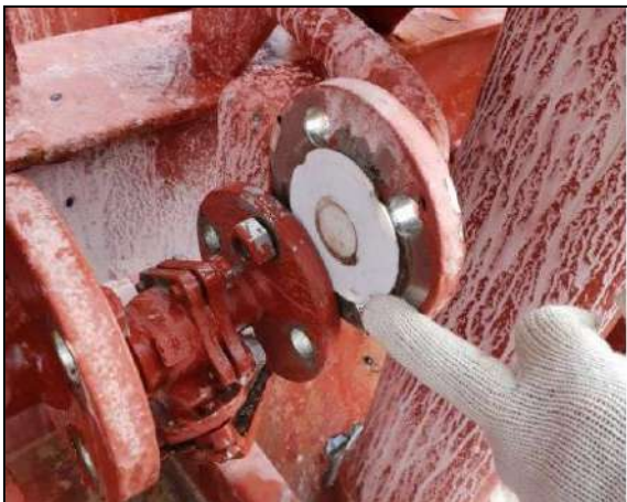
Figure 4: Teflon blank in way of the stripping line
